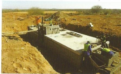
8000l/d WWTP nearing completion
